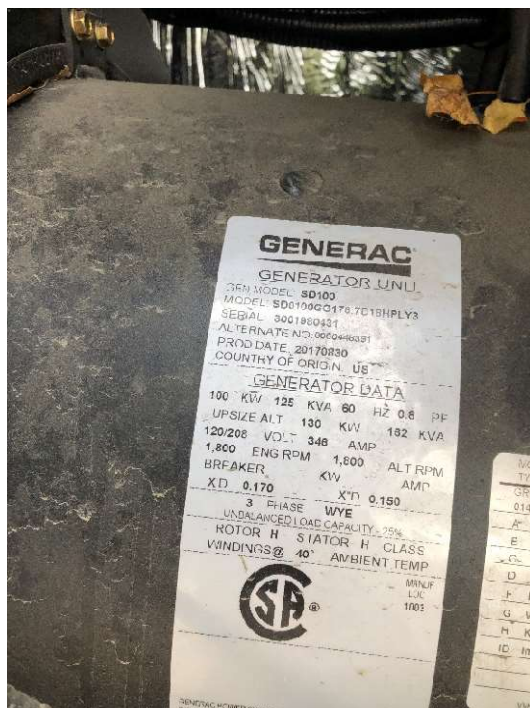
Photo of b/u generator specs
